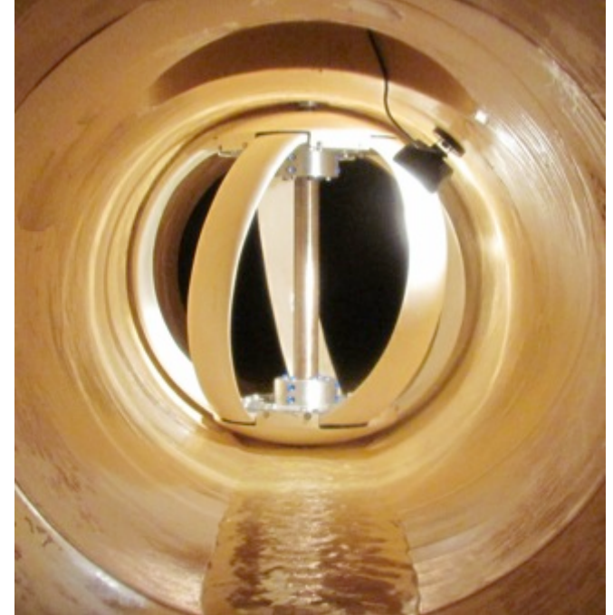
PowerPipe Installed Lemona Pump Station - Riverside, CA
